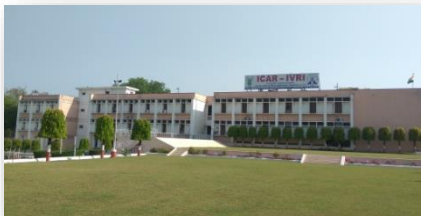
IVRI - Central building
